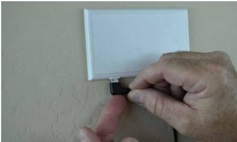
10. Plug the other end of the wire into your tablet. Then, attach the tablet to the S-Mount-P. Route any extra wire behind the tablet so that it is hidden from sight.
